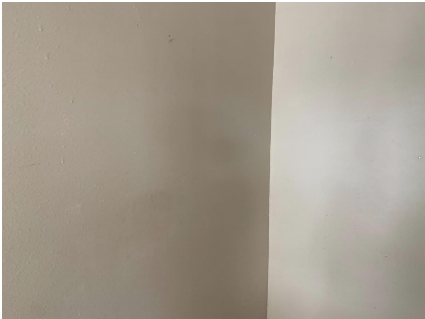
Photograph No. 3 HA-03: White Wallboard with Joint Compound
